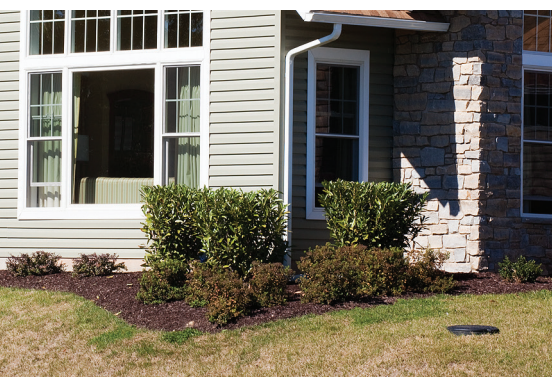
Propane storage can be buried underground with only an inconspicuous service dome showing.
