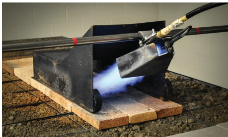
Testing of propane flaming with torch hood
